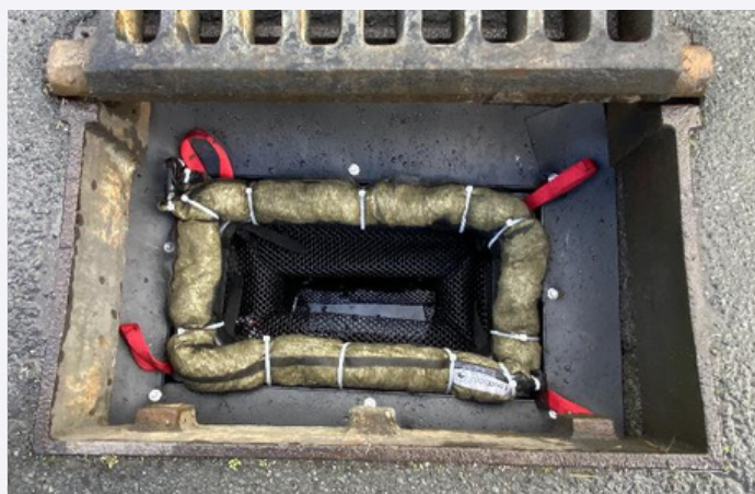
LavaSorb™ boom set up with LittaTrap™ to ensure it absorbs oils and oil-based liquids in the stormwater.
