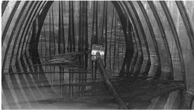
Figure 1— Containment Row shown with high pressure cleaning nozzle
