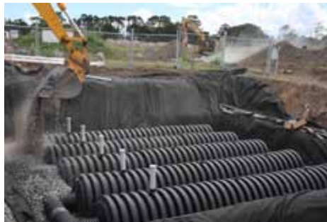
Backfilling chambers with rock
