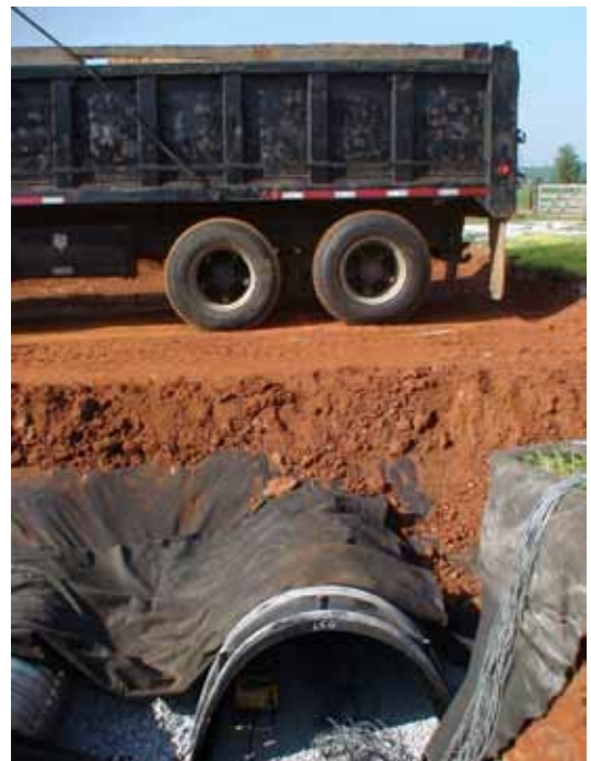
Structural load testing
