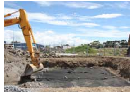
Completed soakage system
