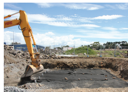
Completed soakage system
