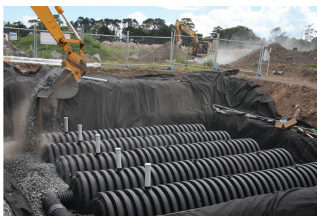
Backfilling chambers with rock
