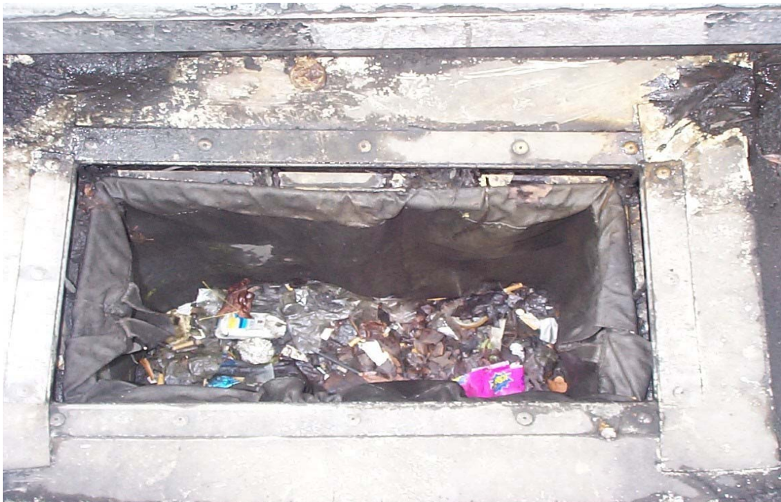
Figure 3 the Enviropod Filter installed
