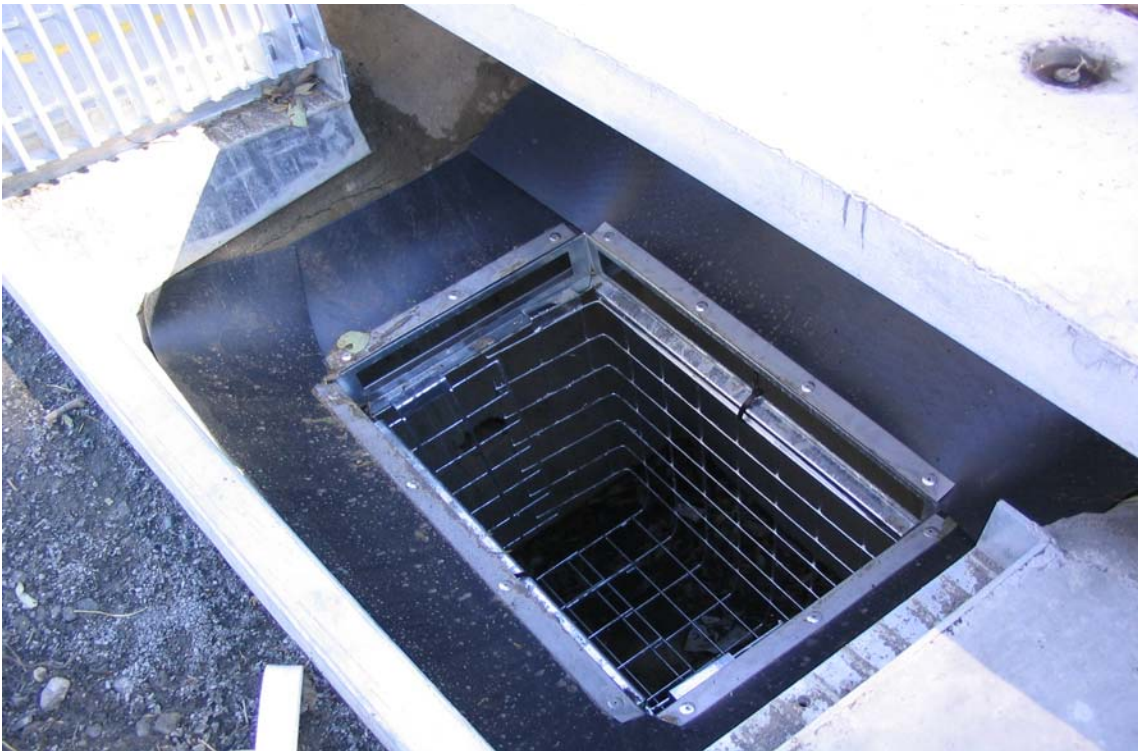
Figure 5 Supporting Frame Work.
