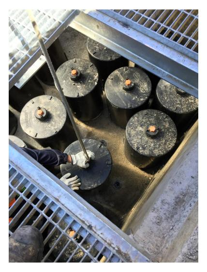
Figure 6: Installing StormFilter Cartridges (Source Stormwater 360, 2016)
