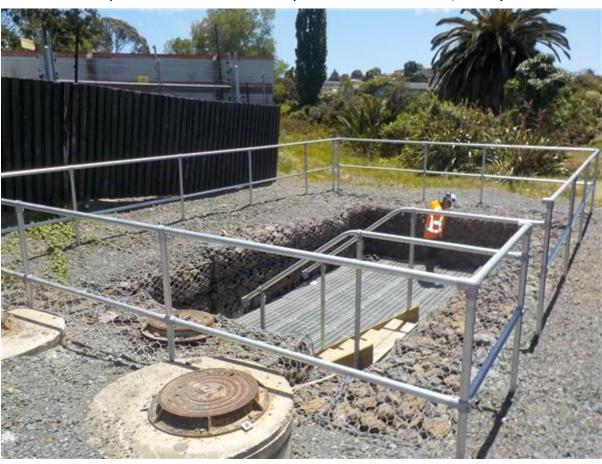
Figure 9: Handrails installed on StormFilter Retrofit (Source: Stormwater360, 2016)
