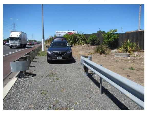
Figure 7: New Guardrail opening. Pre-Sandfilter retrofit (Source: P Mitchell, 2015)
