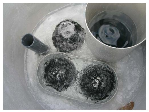
Over the range of the 25 events monitored the treatment system was exposed to varying TSS loads, and a cumulative total of over 75 kg of mass. The TSS was a combination of sediments and organics with a ranging influent concentrations from a low of 25 mg/L to a 2016 Stormwater Conference
